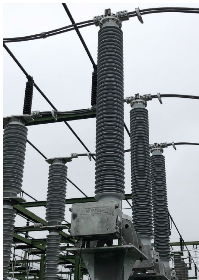
Figure 7: Stationary RC divider for continuous measurement of power quality
