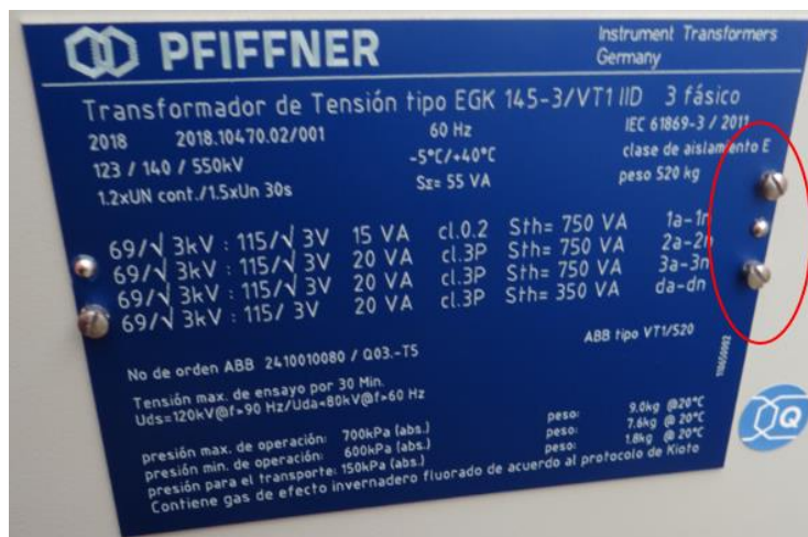
figure 16: sealing for rating plate
