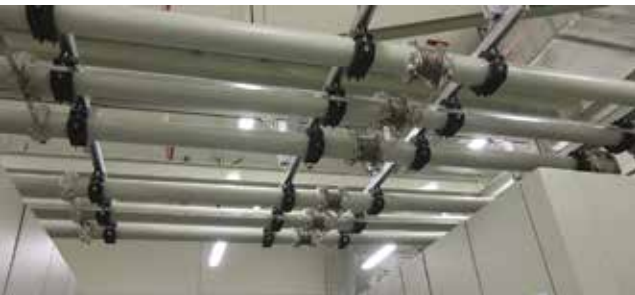
GASLINK® SF 6 insulated busbar system
