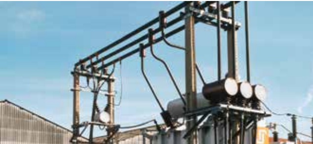
GASLINK® SF 6 insulated busbar system
