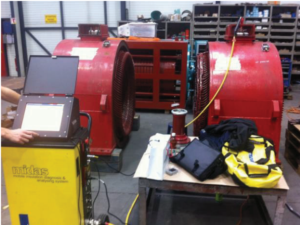
Figure 13: Stator winding with U_n = 5.5 kV.
