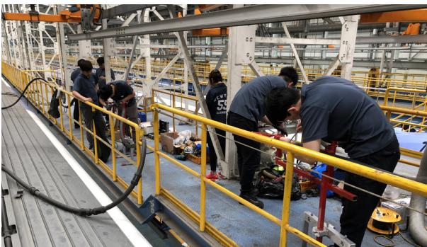
Step 3: On-site execution: Assembly and approval of prototype. Electrical routine test of new installed components on the train. Training of local maintenance personnel. On-site execution of the complete retrofit by ALPHA-ET engineers or by trained local maintenance personnel.
