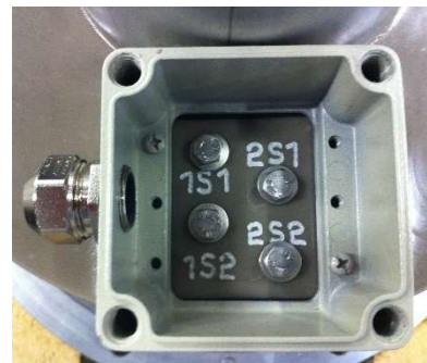
Fig. 8: Example of cable box and nameplate for a current transformer with two cores
